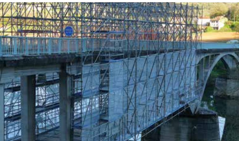
Arcambal bridge (46): mobile scaffolding for renovation works.
