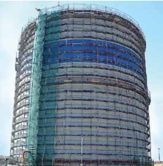
Fos-sur-Mer, GDF site: scaffolding for a Ø 40 m tank.
