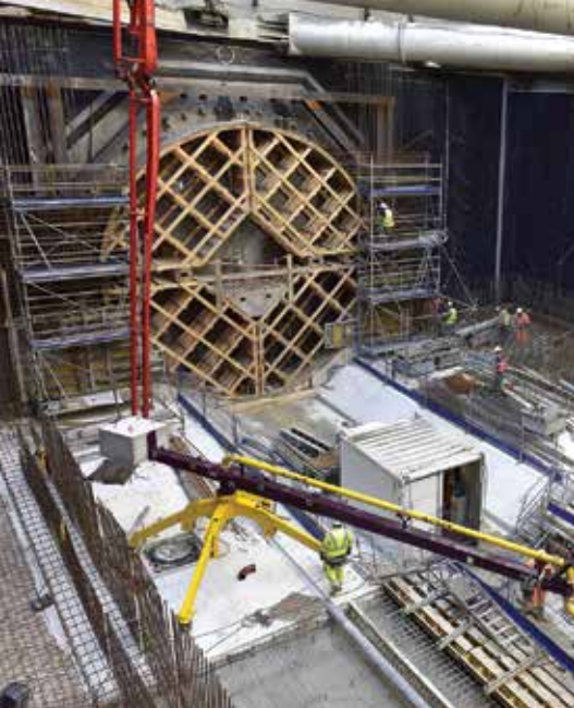
Rennes subway: service scaffolding and shoring at the "Gares" station.
