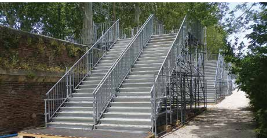
Toulouse: public staircases for extra temporary access during the "Rio Loco" festival.
