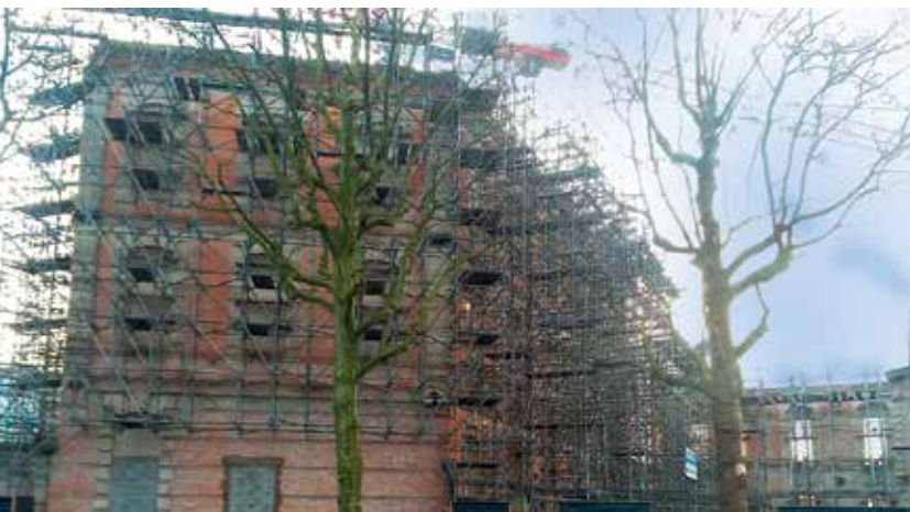
Lille: shoring to the façades of the former Saint-Antoine hospital.
