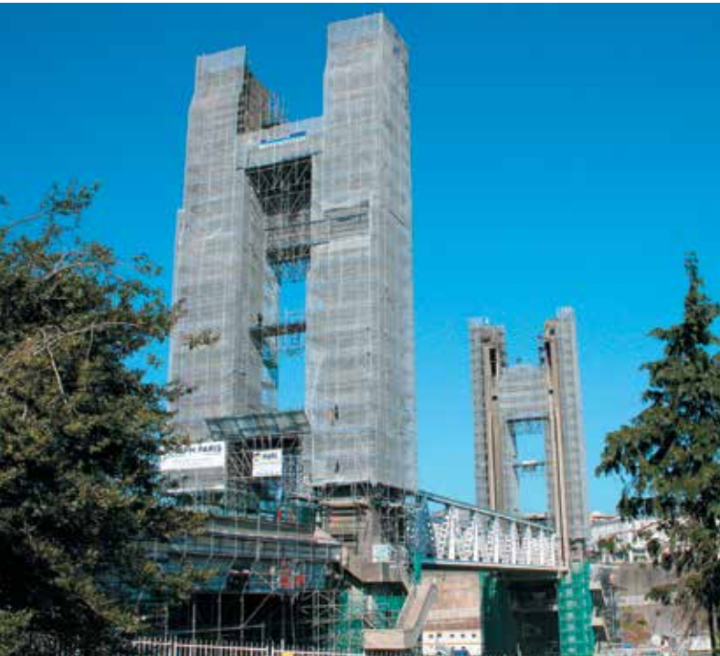
Brest: scaffolding and shoring for refurbishment work on the Recouvrance bridge.
