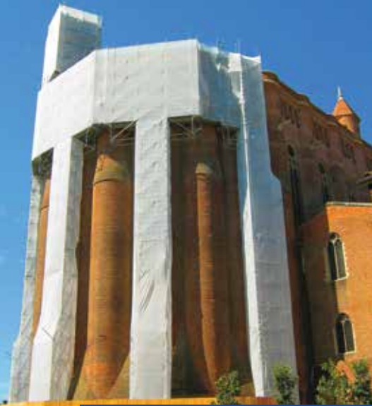
Albi cathedral: scaffolding for the restoration of the coping and stained glass.
