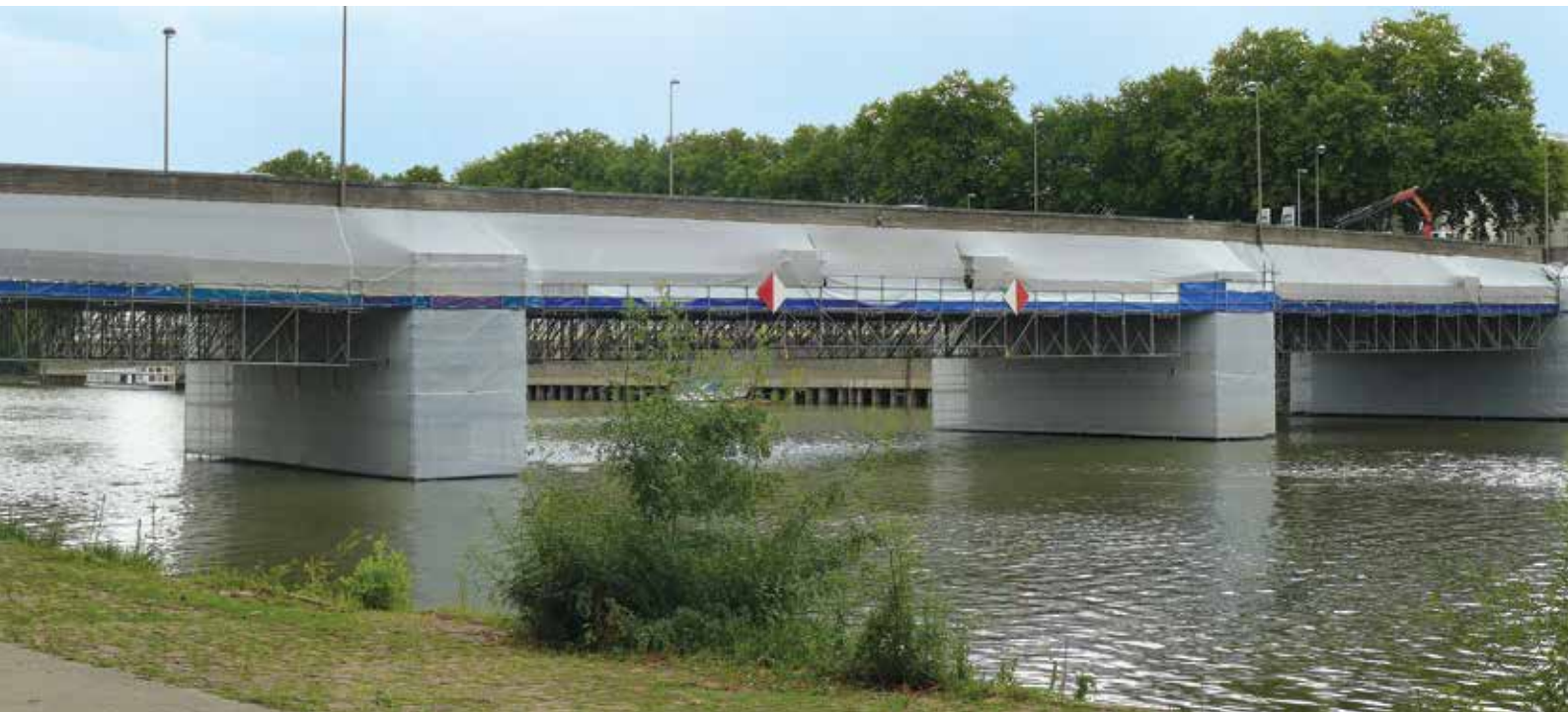
Angers, Haute Chaîne bridge: suspended scaffolding for the renovation.
