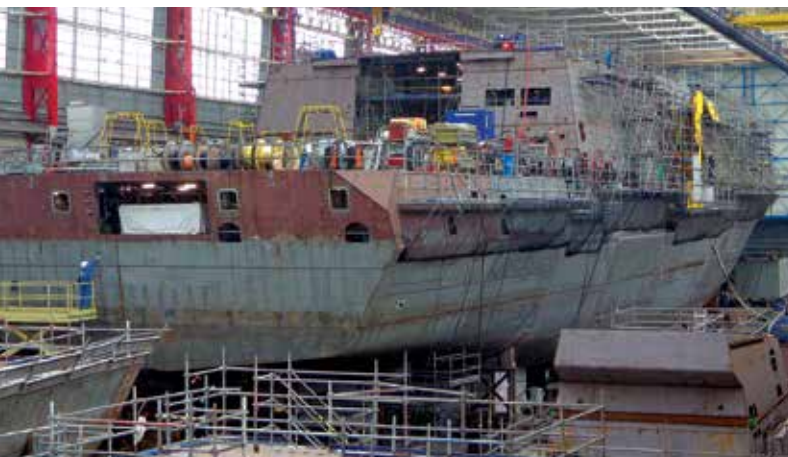
DCNS Brest: scaffolding for the construction of FREMM frigates.
