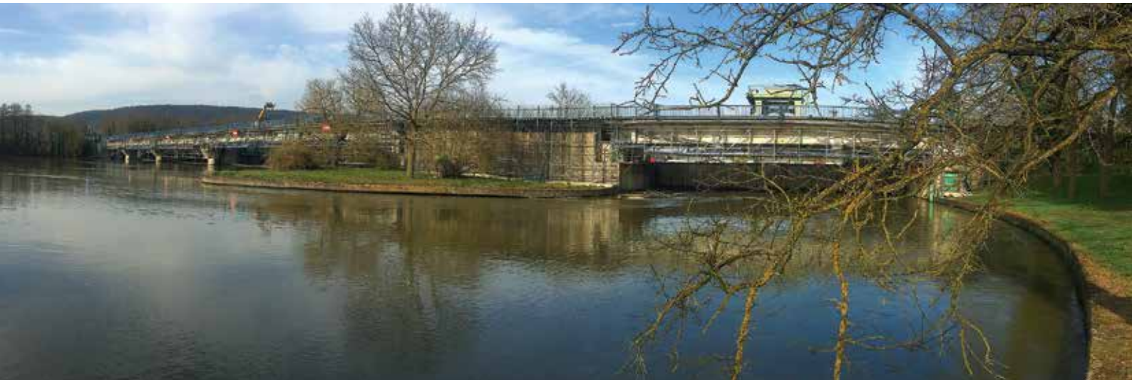
Jouy-aux-Arches, dam: suspended scaffolding and public walkways.
